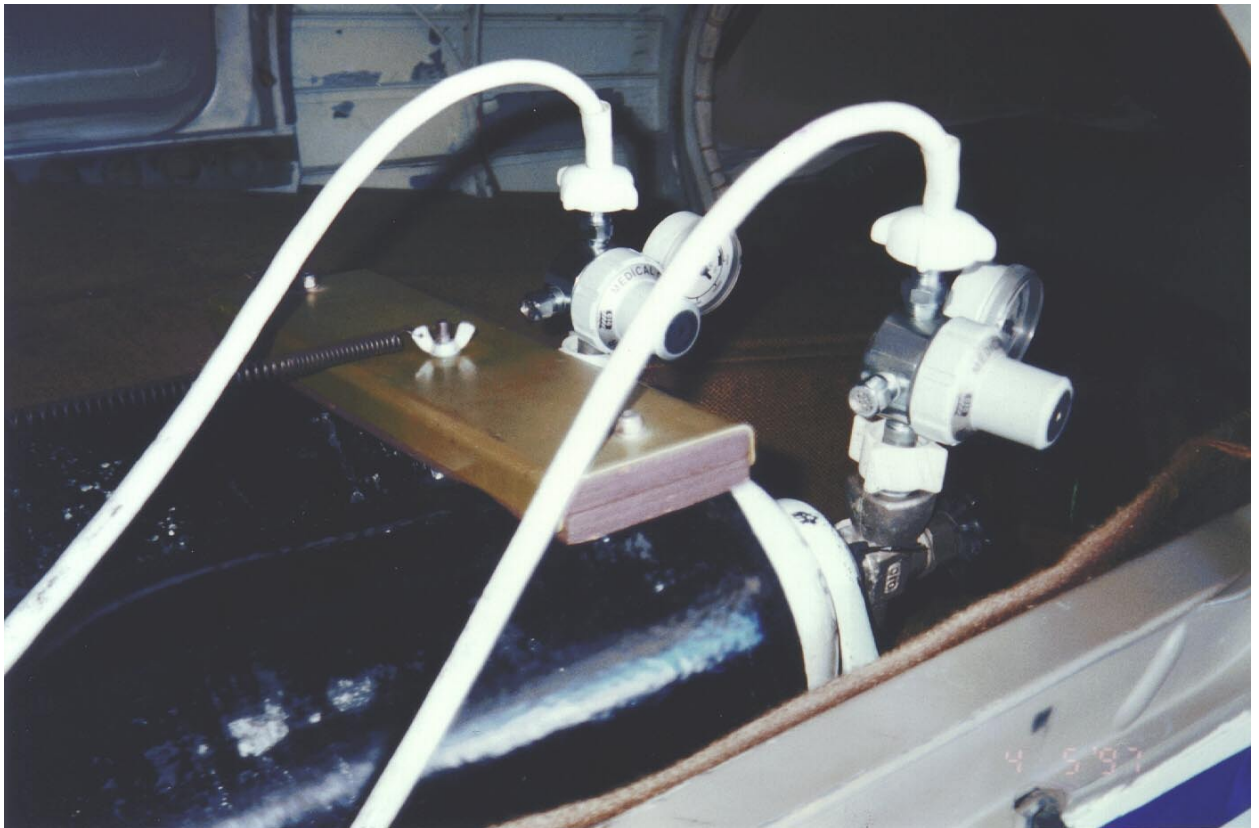
A fixed wing aircraft was found with an unsafe installation of oxygen bottles and hoses in the nose locker. There was no way to turn these bottles off from inside the aircraft.
