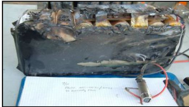
36-cell lithium-ion battery pack with thermal damage.
