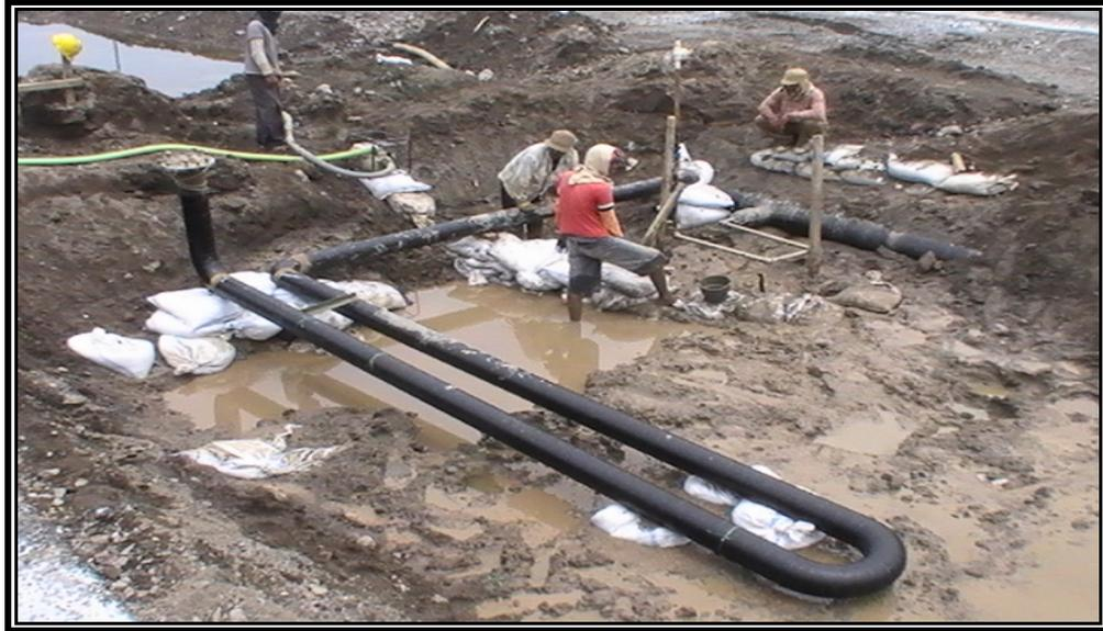
*Figure 5 – A photo taken during the tie-in process*
