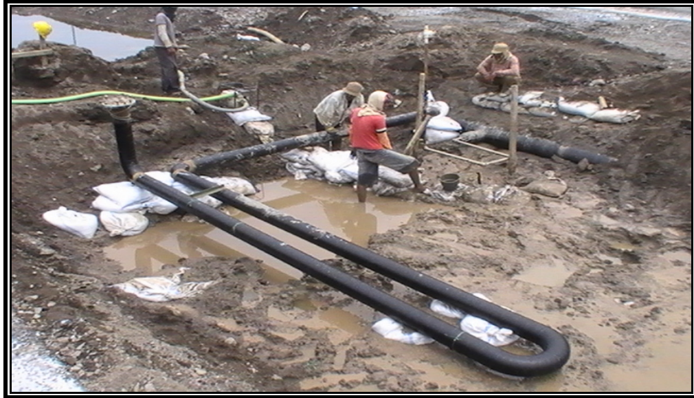
Figure 5 – A photo taken during the tie-in process
